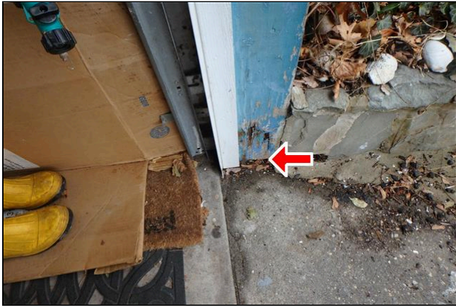
5.2 Item 1(Picture) The inspector noticed rot on the door jamb on base of the garage door.
