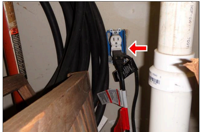
13.3 Item 4(Picture) The sewage ejection pump is not GFCI protected
