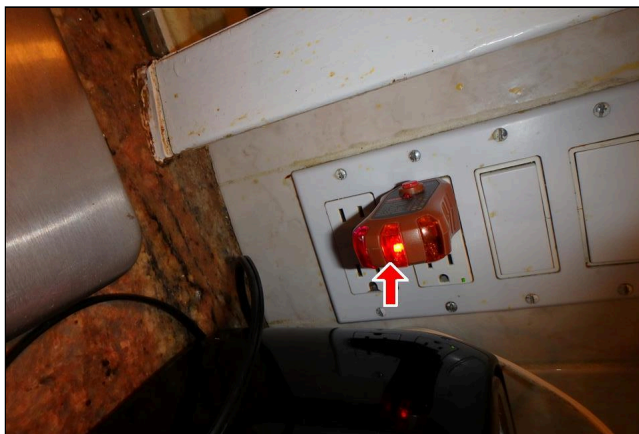
13.3 Item 24(Picture) There are ungrounded receptacles in the kitchen
