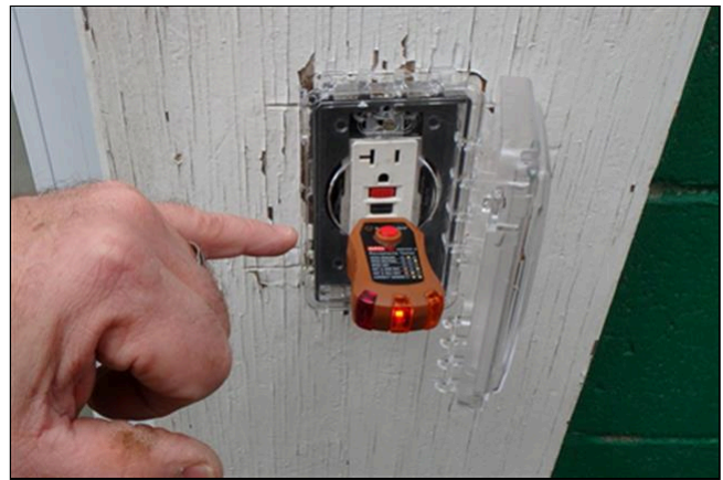
13.3 Item 13(Picture) The GFCI receptacle on the exterior by the patio door is defective
