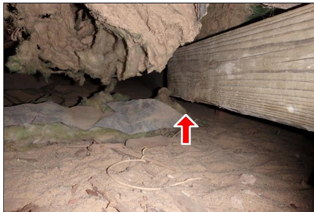
11.3 Item 2(Picture) The girder under the living room is not supported (seen from the wine cellar)
