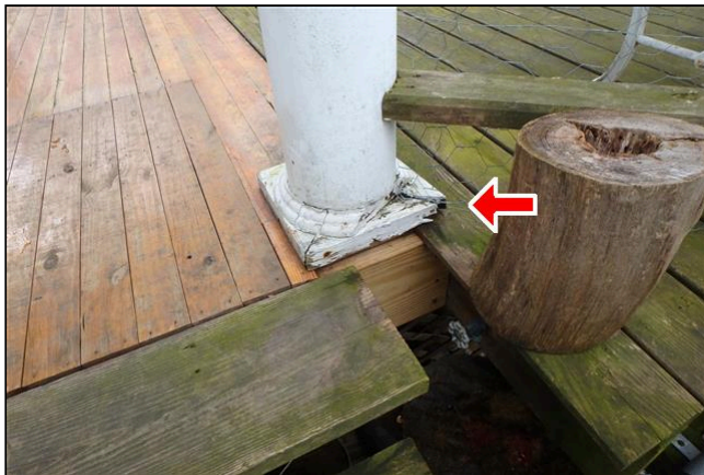
3.0 Item 10(Picture) The column on the north deck is rotted
