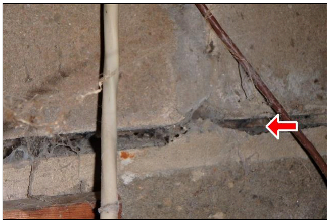
11.0 Item 1(Picture) The north foundation wall in the guest house is failing (2) Cottage
