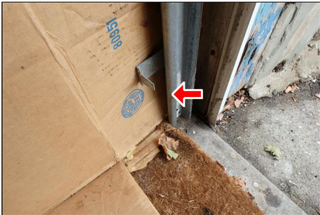
5.3 Item 1(Picture) The garage door opener was operational but does not have safety beams
