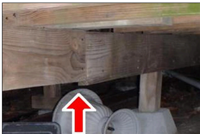
4.3 Item 3(Picture) The girder on the pool deck is separating at the seam due to lack of support
