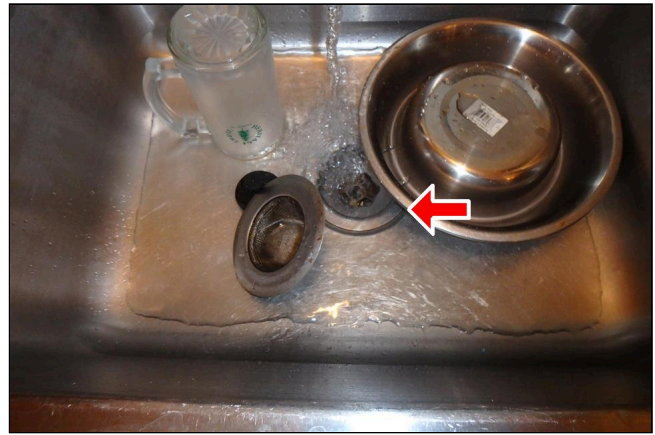
12.0 Item 6(Picture) The inspector noticed that the kitchen sink syphons when draining from poor ventilation.
