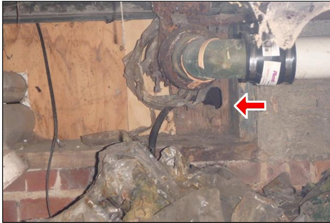
3.0 Item 8(Picture) There are opening in the plywood in the basement window allowing infestation
