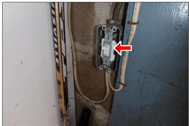
13.3 Item 2(Picture) There is missing cover plates for the switches and outlets scattered through out the house
