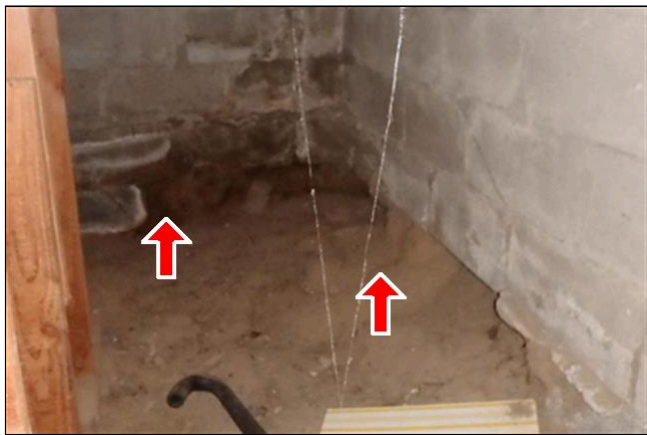
11.0 Item 2(Picture) The foundation in the southeast corner of the crawlspace has no footing and is being compromised
