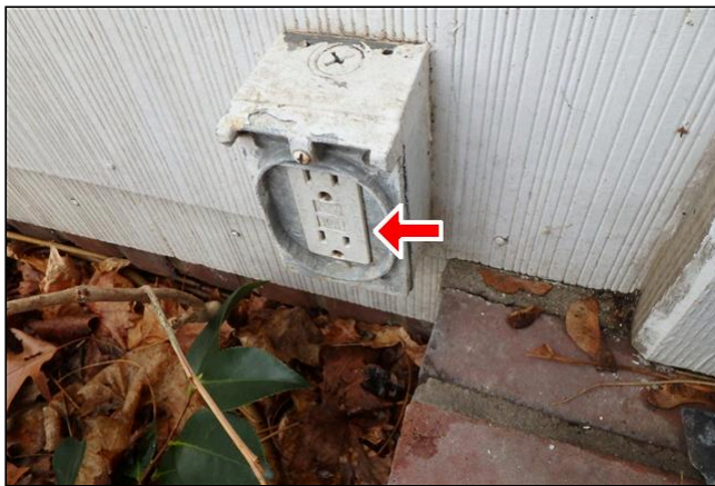
13.3 Item 19(Picture) The exterior GFCI receptacle is defective to the left of the front entrance and is missing a cover
