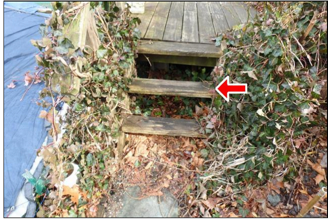
4.2 Item 2(Picture) The stairs on the pool are deteriorated and missing a railing
