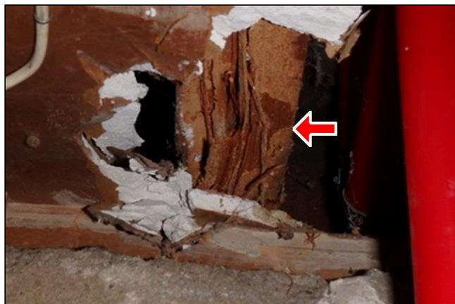
11.8 Item 1(Picture) The floor joists in the guest house on the north wall have been effected by termites
