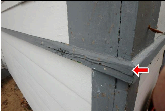
3.0 Item 5(Picture) Deteriorated trim on the south east corner of the house
