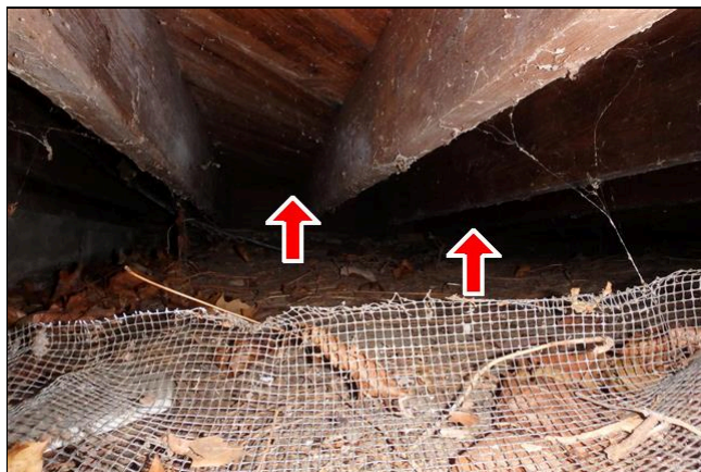
15.1 Item 1(Picture) The floor of the office is not insulated or protected from weather or infestation
