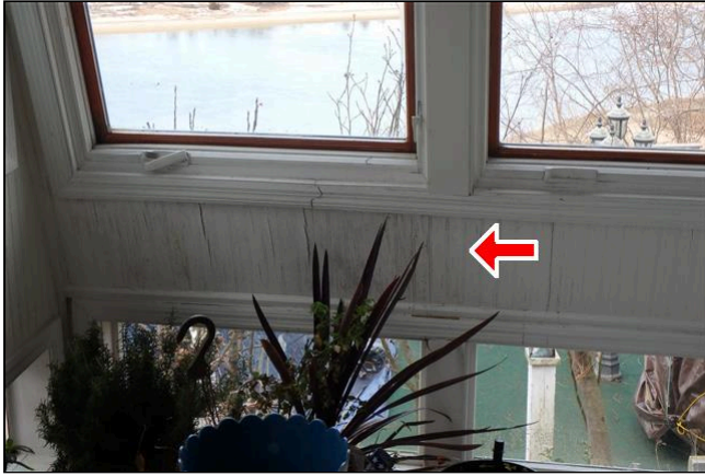
3.5 Item 5(Picture) There is an active leak in the bathroom windows on the 1st floor facing north
