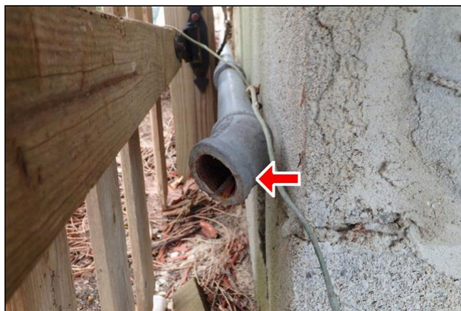
6.3 Item 1(Picture) There is an open gas line on the east side of the exterior missing a cap
