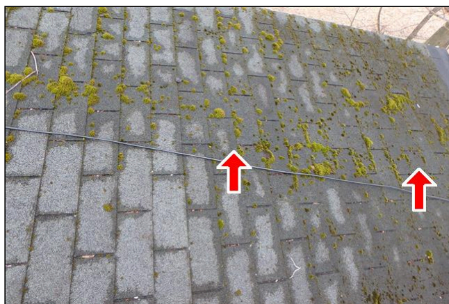
2.5 Item 1(Picture) The inspector noticed moss/lichen growth on the roof and black algae streaks
