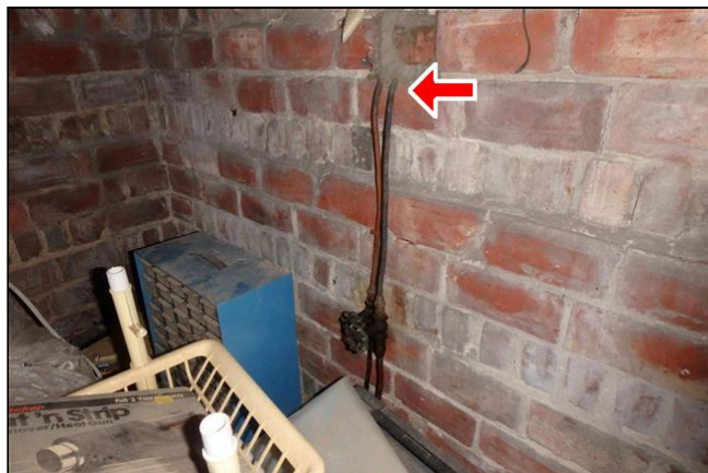
6.0 Item 1(Picture) The inspector noticed signs of a buried oil tank and recommends obtaining a abandonment certificate
