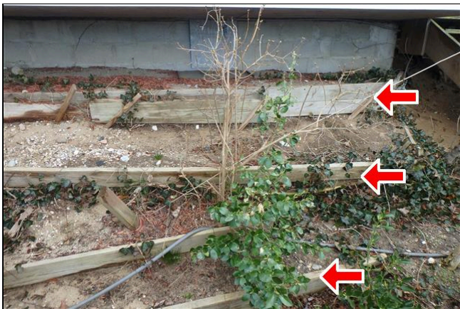
1.3 Item 5(Picture) The retaining walls on the north side are deteriorated
