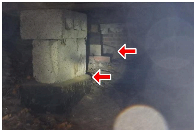
4.3 Item 1(Picture) The porch is not properly supported and requires further evaluation
