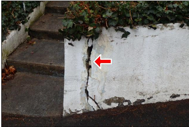
1.3 Item 1(Picture) Retaining walls are deteriorated
