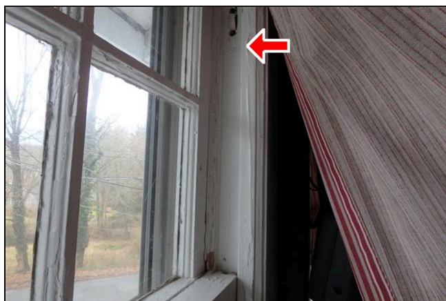
3.5 Item 1(Picture) The inspector noticed broken window sash cords scattered around.
