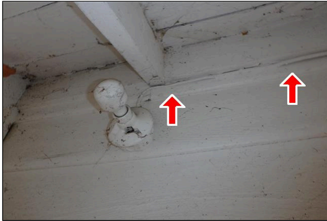
13.3 Item 5(Picture) Exposed romex on the exterior by the entrance door
