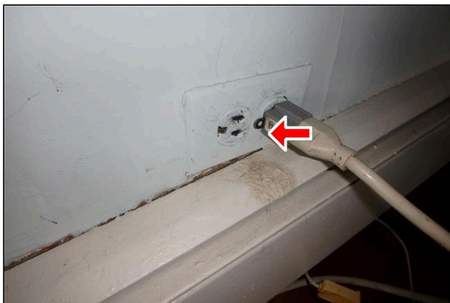
13.3 Item 23(Picture) There are painted over outlets scattered throughout that should be replaced
