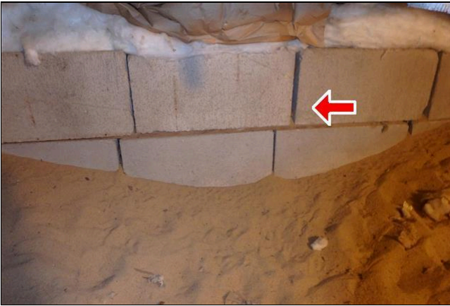
11.0 Item 3(Picture) The foundation on the north wall in the wine cellar are not properly constructed
