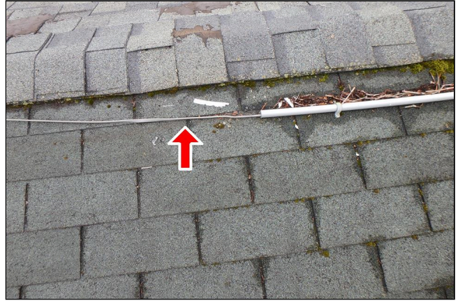
13.3 Item 18(Picture) There is exposed romex wire on the garage roof
