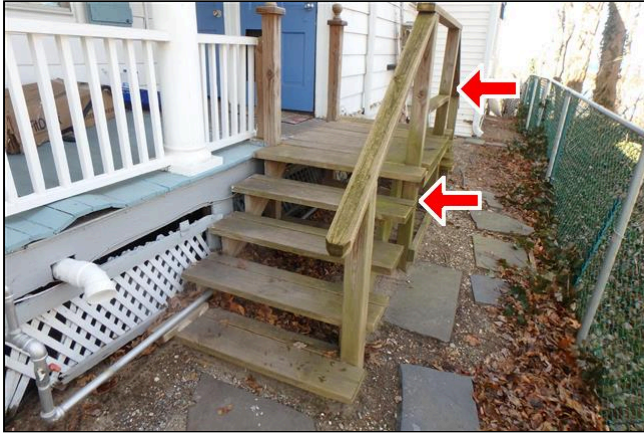
4.2 Item 5(Picture) The inspector noticed that the railing baluster spacing is beyond the current recommended 4 inch standard on the east side stairs
