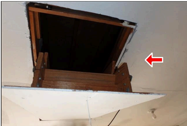
5.0 Item 2(Picture) The installation of wood attic stairs is a breach in the fire rock
