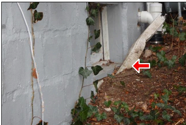
3.6 Item 1(Picture) Installing window wells on the guest house to create the 6 inch soil clearance is recommended.
