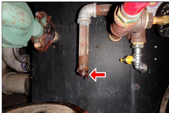
14.0 Item 2(Picture) leaking TPS valve
