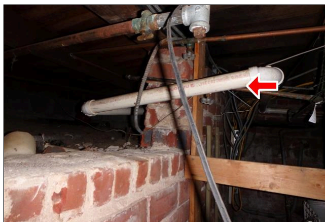
12.0 Item 10(Picture) Washing machine drain pitched backwards
