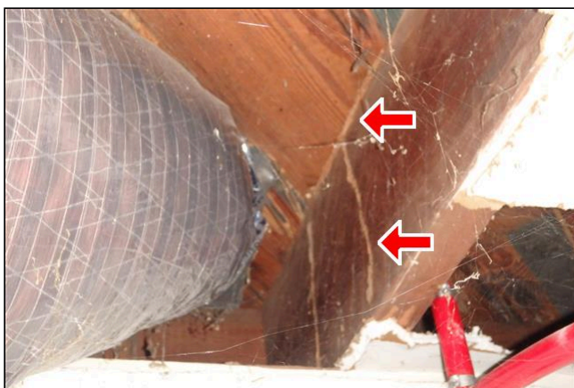
11.7 Item 1(Picture) The inspector noticed termite activity in the guest house floor joists on the north wall
