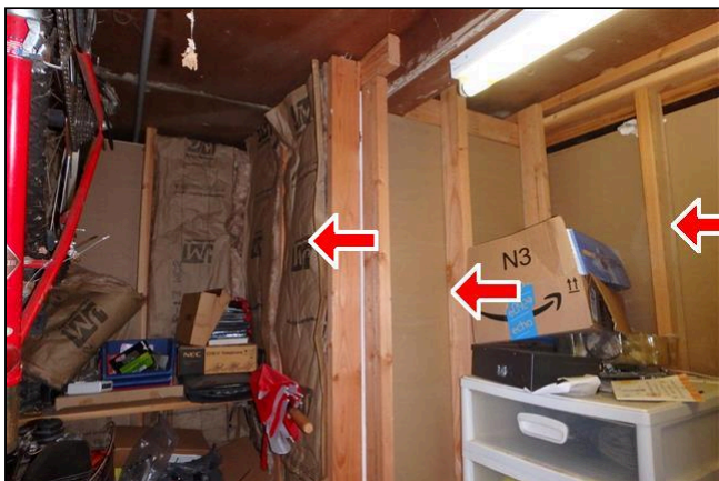
7.1 Item 1(Picture) Backwards and missing insulation in the apartment walls in the apartment walls
