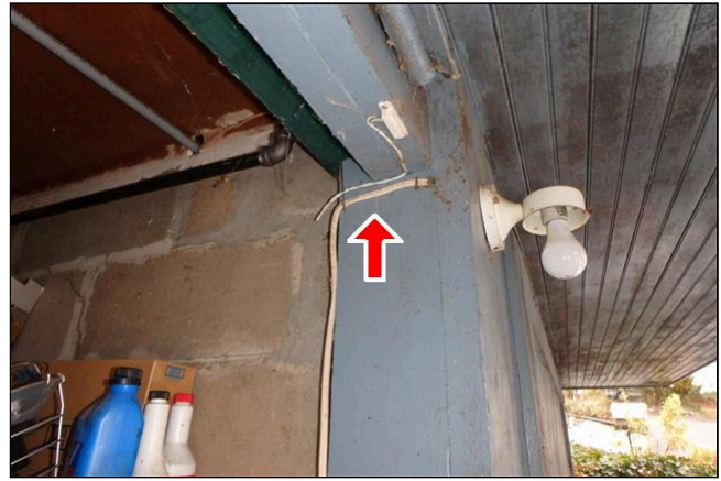
13.3 Item 6(Picture) Exposed romex by the garage door entrance
