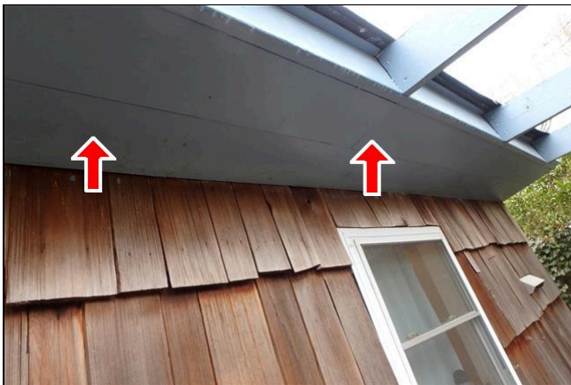
3.1 Item 1(Picture) The inspector noticed a lack of soffit vents around the house.
