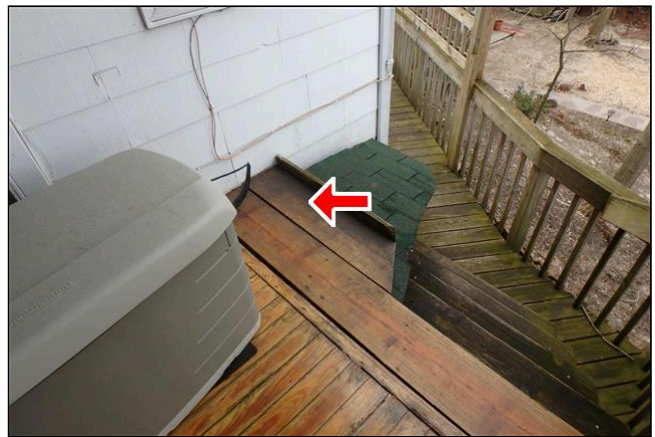
4.2 Item 4(Picture) Missing railing on the north west corner of the deck
