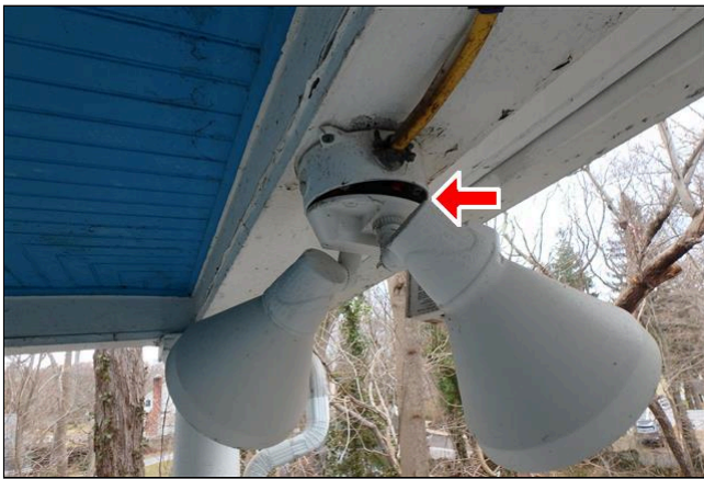
13.3 Item 21(Picture) The spot light on the porch is not properly secured
