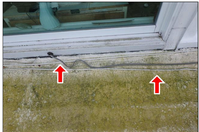
13.3 Item 16(Picture) There is a romex wire on the north lower roof outside of conduit and not secured
