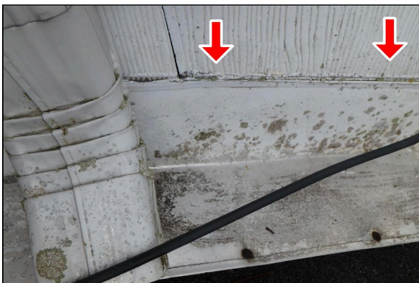
2.2 Item 1(Picture) The flashing on the upper west wall is installed incorrectly.
