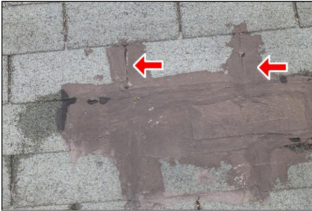
2.0 Item 1(Picture) There are some tared repairs to the roof that are deteriorated
