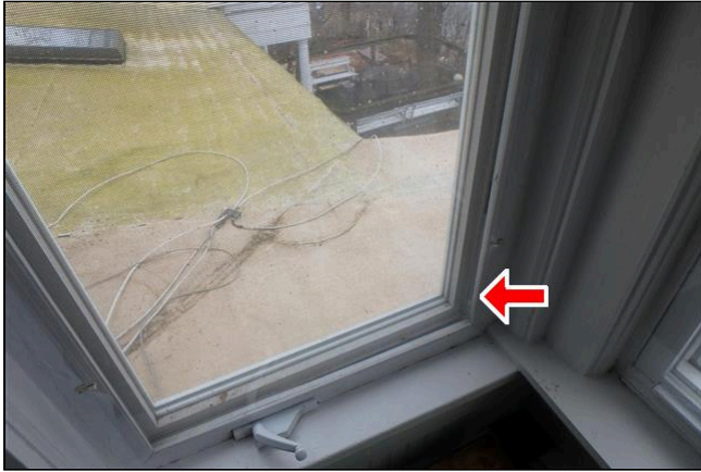
3.5 Item 2(Picture) The casement window on the west side will not lock
