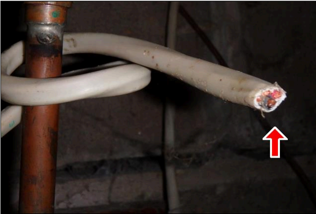
13.3 Item 1(Picture) There are terminated wires in the garage outside of a junction box
