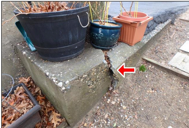
1.3 Item 4(Picture) The retaining wall to the east side is deteriorated
