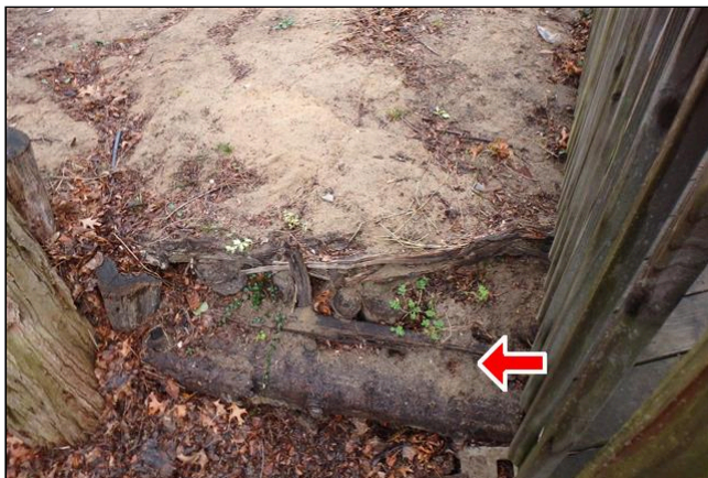
1.3 Item 3(Picture) The wood retaining wall is rotted to the left of the deck
