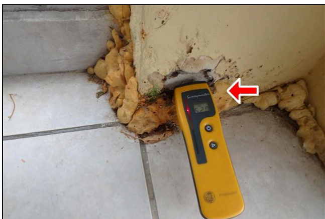
7.1 Item 2(Picture) There is an active water leak at the base of the patio door on both walls.
