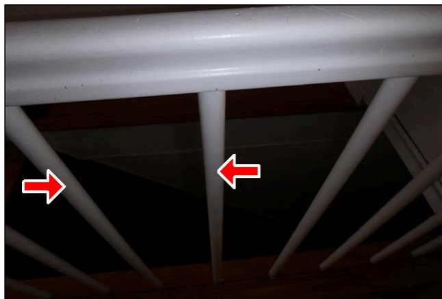
7.3 Item 1(Picture) The interior hand rail and baluster spacing is beyond the current 4 inch requirement.
