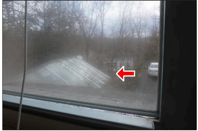
3.5 Item 4(Picture) The inspector noticed broken window seals scattered throughout the house
