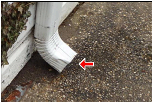
2.4 Item 1(Picture) The gutter leaders are depositing water at the base of the foundation on all the houses.
