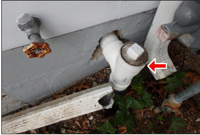
12.0 Item 1(Picture) There is no presents of a fresh air intake on the septic system
