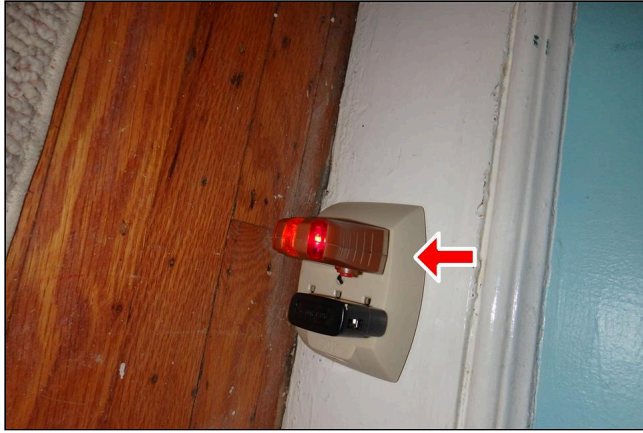
13.3 Item 9(Picture) The inspector noticed hot and neutral reversed receptacles scattered through out the house
