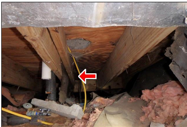
11.3 Item 1(Picture) The floor joist in the crawlspace under the bathroom on the north 1st floor has been compromised
