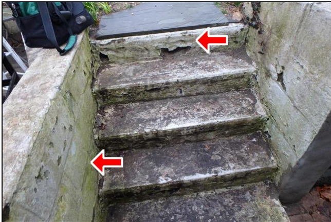
1.1 Item 1(Picture) The north steps are deteriorated and missing a handrail
