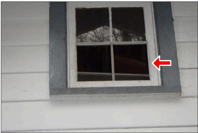
3.0 Item 4(Picture) There is no glass present in the attic window
