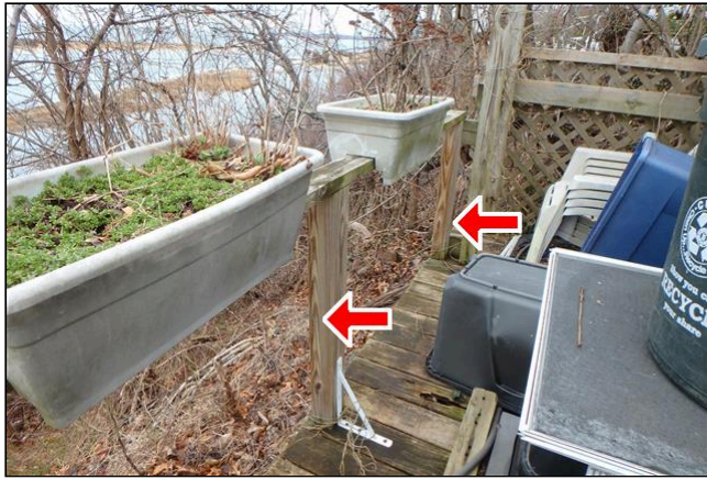
4.2 Item 1(Picture) The inspector noticed that the railing baluster spacing is beyond the current recommended 4 inch standard.
