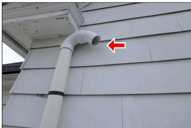
12.0 Item 7(Picture) There is a plumbing vent stack on the west side of the house that is too close to the structure and window openings
