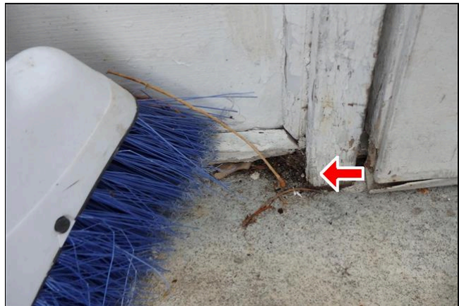
3.0 Item 7(Picture) The front entry door trim is rotted at the base
