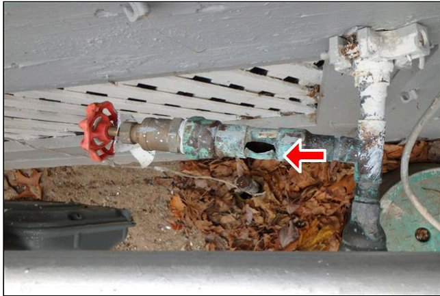
12.1 Item 3(Picture) The water faucet supply line burst on the east side of the exterior
