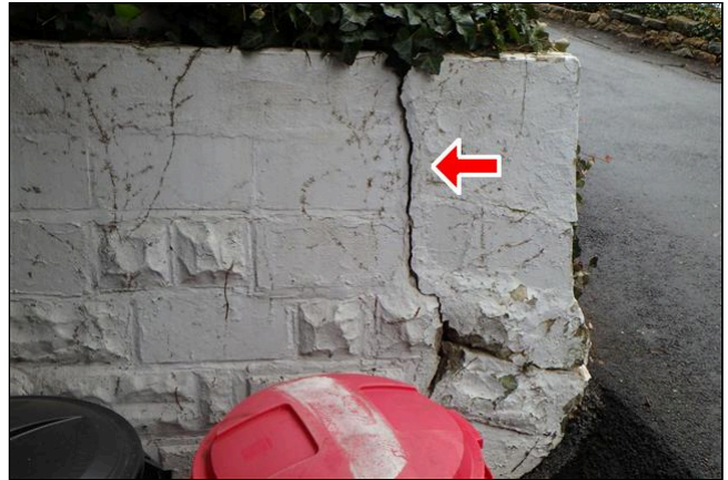
1.3 Item 2(Picture) Offset cracks in the retaining wall
