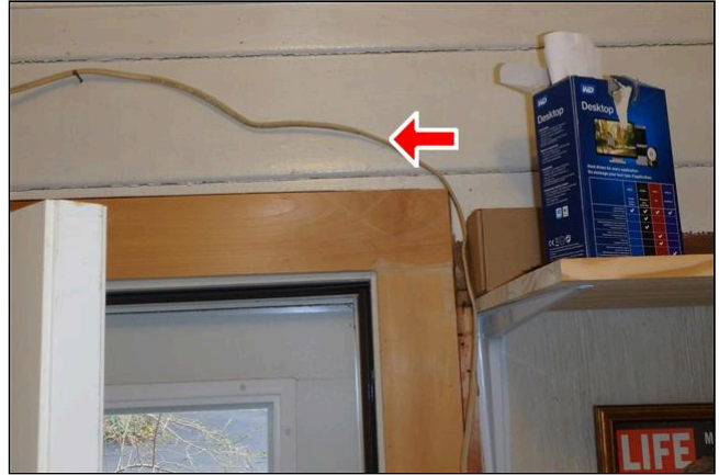
13.3 Item 10(Picture) Exposed romex wire in the office area
