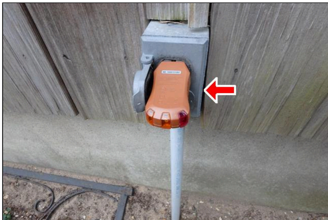
13.3 Item 12(Picture) There is no power at the exterior receptacle on the north wall
