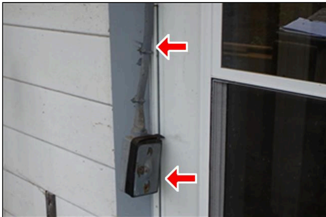
13.3 Item 7(Picture) Exposed romex and unsecured light switch by the exterior front door
