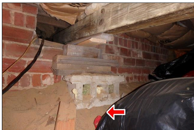
11.2 Item 1(Picture) There are no footings under many of the columns in the wine cellar
