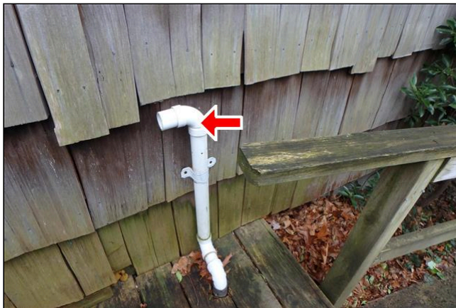
12.0 Item 5(Picture) There is a plumbing vent on the east side of the cottage that origin is unknown
