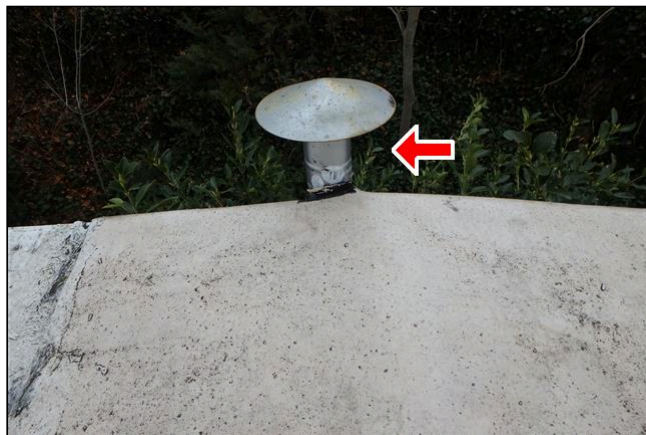
14.4 Item 1(Picture) The hot water heater flu is too close to the roof
