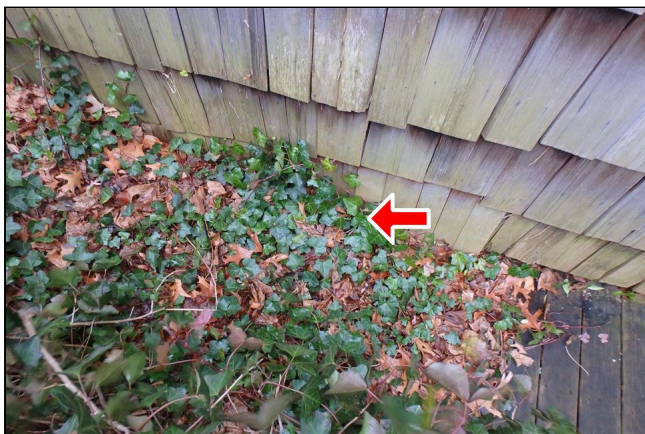
3.7 Item 4(Picture) It is recommended that the soil be 6 inches below the siding to prevent damage to the structure and inspect infestation on the cottage and main house
