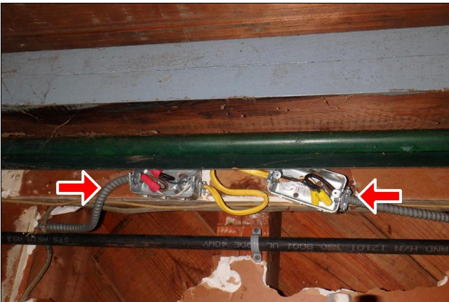
13.3 Item 3(Picture) Open junction boxes in the garage
