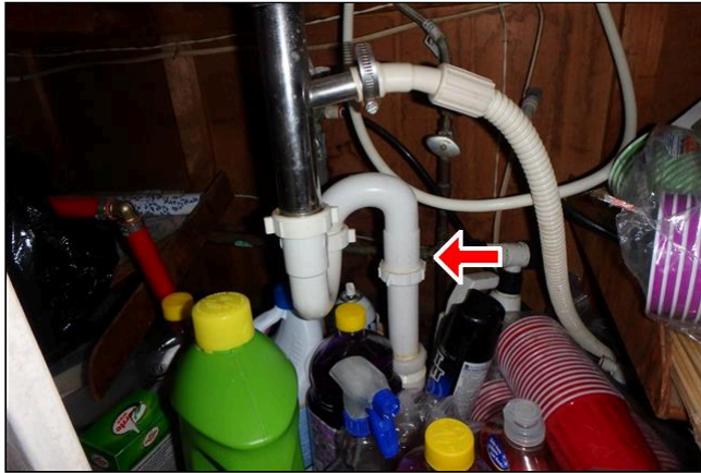
12.0 Item 3(Picture) The inspector noticed a "S" trap under the kitchen sink
