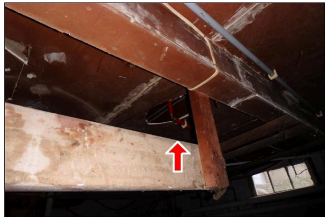
5.0 Item 1(Picture) The garage in the guest house is missing fire retardant sheet rock in sections in the garage
