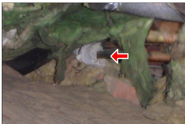
11.9 Item 1(Picture) There is evidence of pipe wrap known to contain asbestos in the the crawl space
