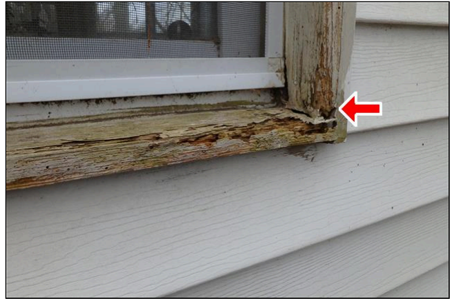
3.0 Item 9(Picture) There is scattered trim rotted around the house
