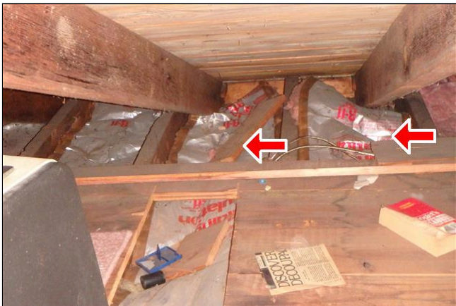
15.0 Item 1(Picture) The insulation was installed backwards with the vapor barrier facing away from the heated sections of the house
