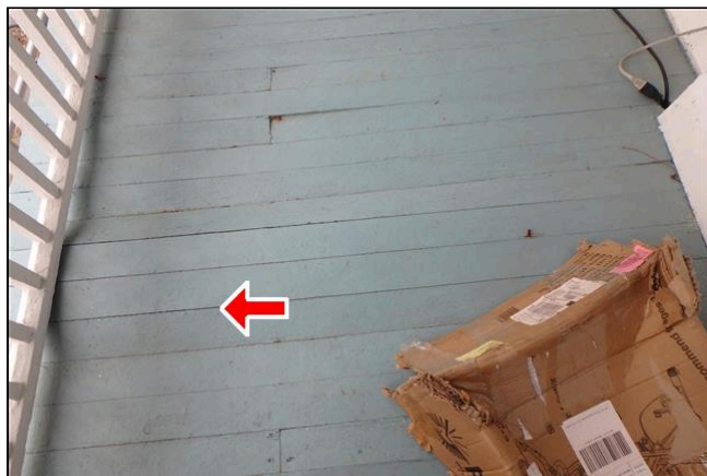
4.1 Item 1(Picture) There are buckling and rotted deck boards on the front porch
