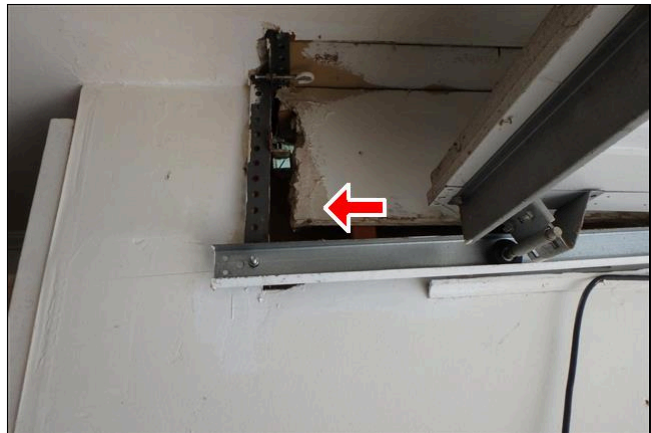
5.0 Item 3(Picture) There are holes in the sheetrock in the garage
