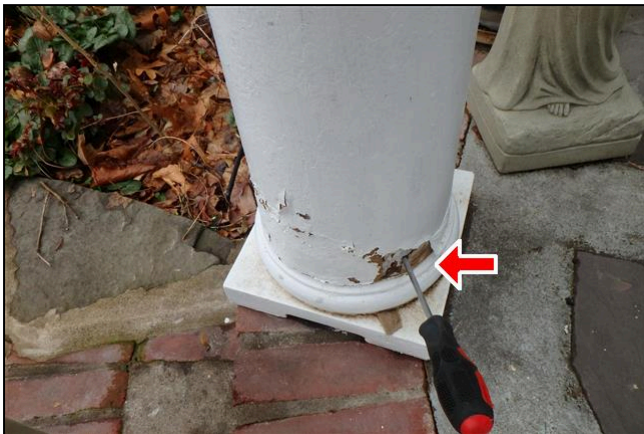
3.0 Item 6(Picture) The columns by the front entrance are deteriorated at the base
