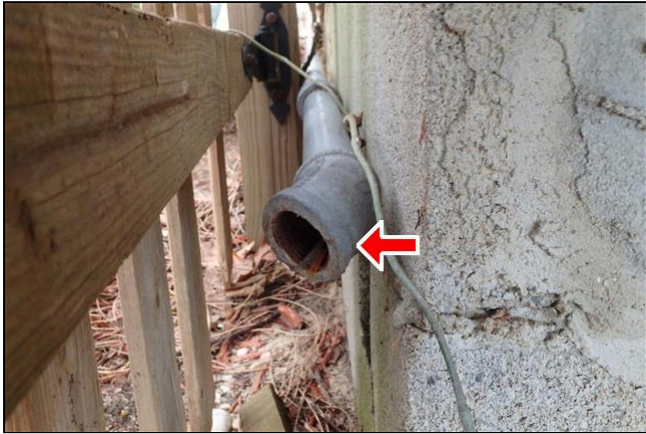
6.3 Item 1(Picture) There is an open gas line on the east side of the exterior missing a cap 6.3 Item 2(Picture) The inspector noticed the presence of corrugated stainless steel tubing (CSST) used for gas service on the boiler.
