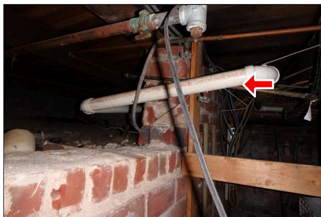
12.0 Item 10(Picture) Washing machine drain pitched backwards
