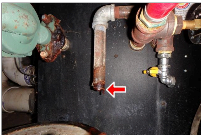
14.0 Item 2(Picture) leaking TPS valve
