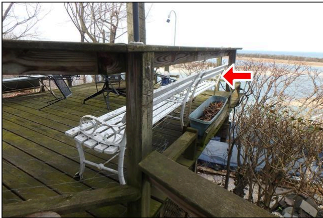
4.2 Item 3(Picture) The inspector noticed that the railing baluster spacing is beyond the current recommended 4 inch standard.
