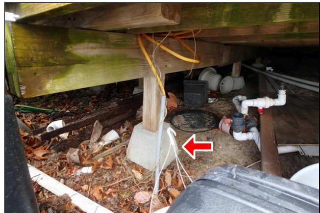
4.3 Item 2(Picture) The pool deck has no footings and is improperly supported
