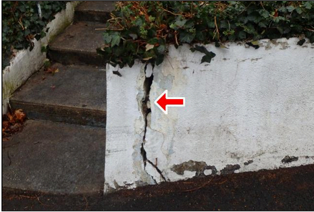
1.3 Item 1(Picture) Retaining walls are deteriorated
