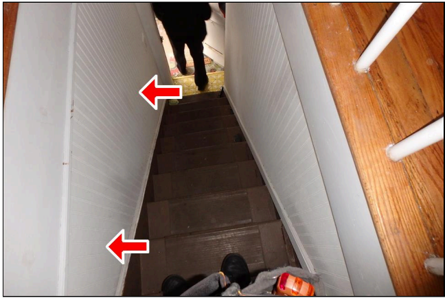
7.3 Item 2(Picture) There is also no handrail present on the stairway.
