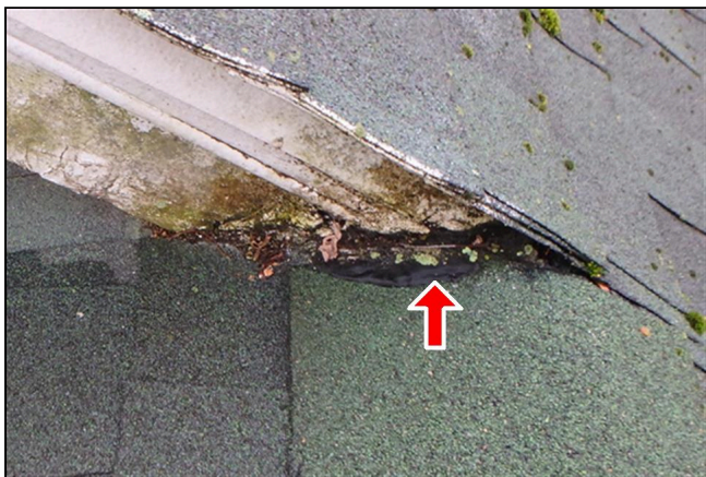
3.0 Item 1(Picture) There is deteriorated trim scattered around the house
